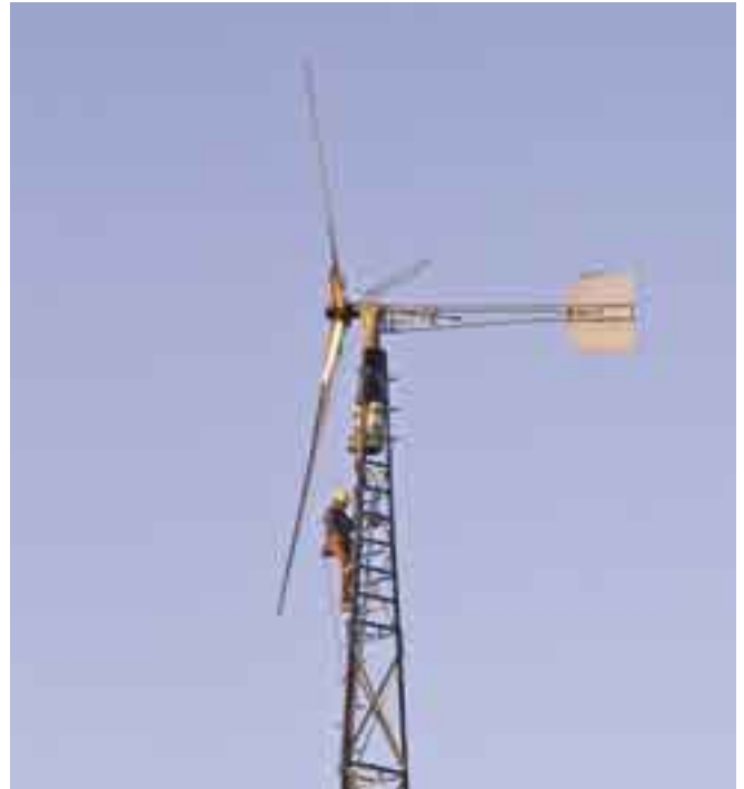
Mike Dooraghi of the SWI team makes the long 120-foot climb up to the Jacobs for some maintenance.
